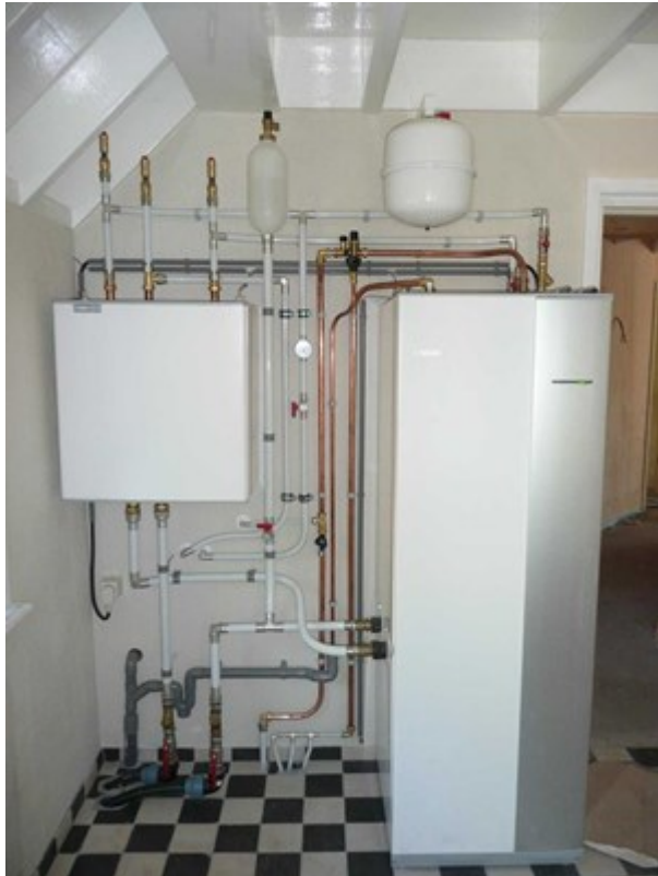
Afb. 9.30 Water-waterwarmtepomp
